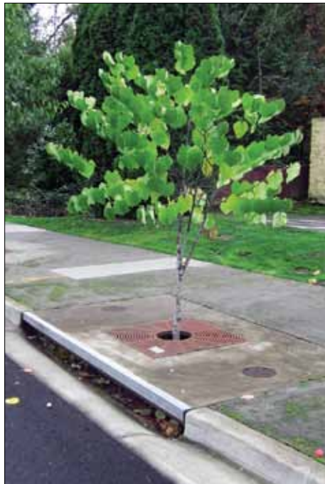
Existing Filterra Unit on 9th Avenue SE
